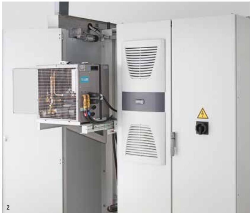
1 Critical components are stored safely to keep them out of the rough environment and prevent damage which increases the system uptime. 2 Easy maintenance with the extendable cooler unit
